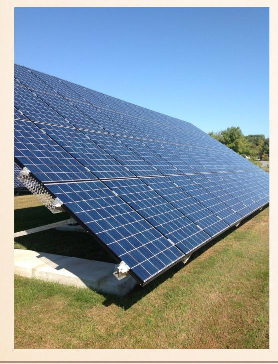
4 arrays 224 panels 12,096 cells 64 kW system
